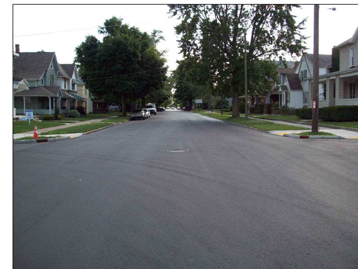
As mandated by the United States Government, whenever the City repaves a street it MUST replace all handicap ramps at each intersection and bring them up to current ADA standards. Current ADA standards call for Detectable Warning Devices which are the yellow or red plates that you see within the sidewalk. These are to signal people that they are at the street.
