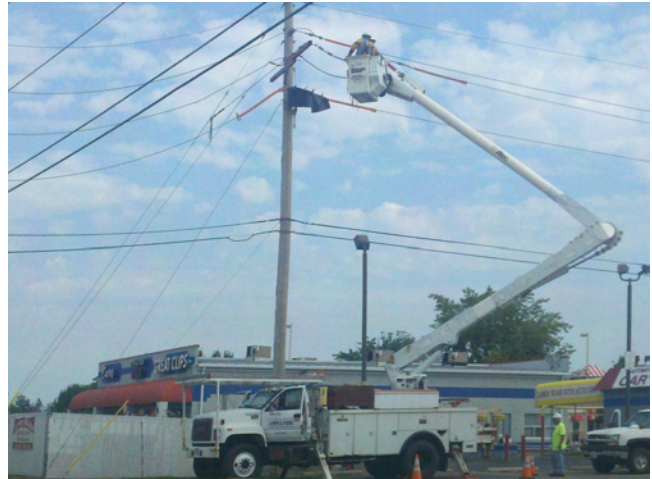
Electrical lines being installed north of the bypass
