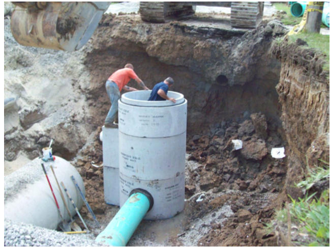
Combined sewer separation project on Division Street
