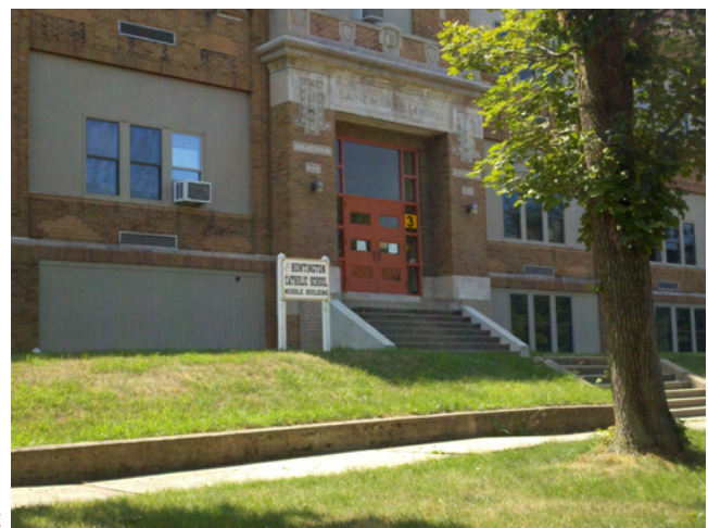
Huntington Catholic School Middle Building
