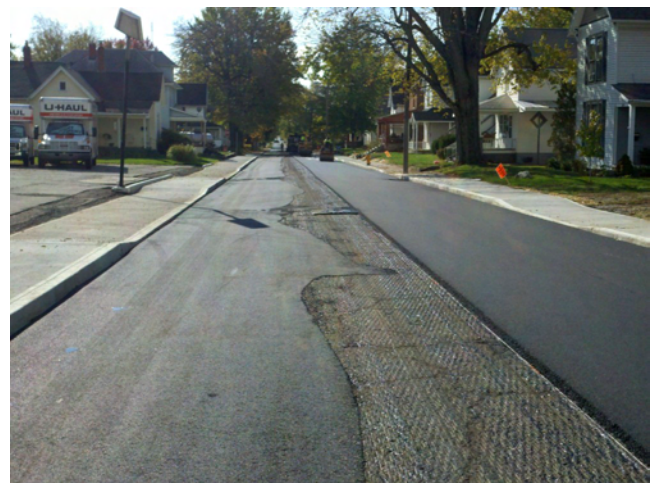
Salamonie Avenue, a Collector Street gets repaved
