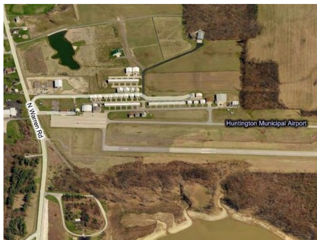
Huntington Municipal Airport
