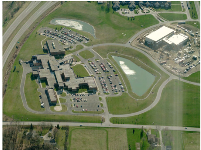
The Parkview Huntington Hospital Campus as of 2008
