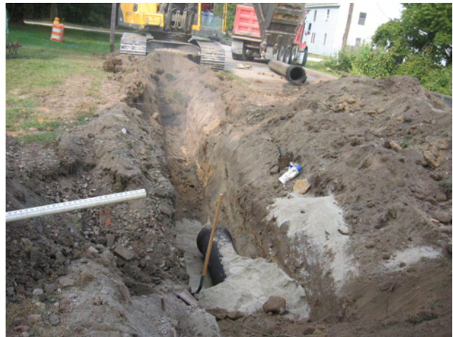
E. State Street water main extension to service Park 24
