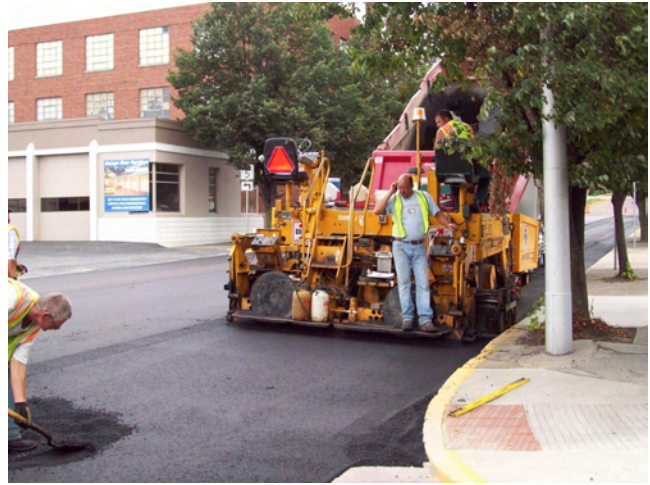
Street paving project on Warren Street near downtown
