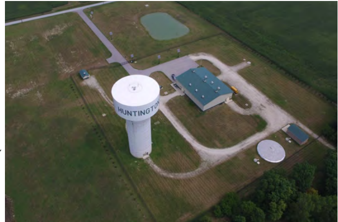
Huntington's North Water Plant on CR 600 N
