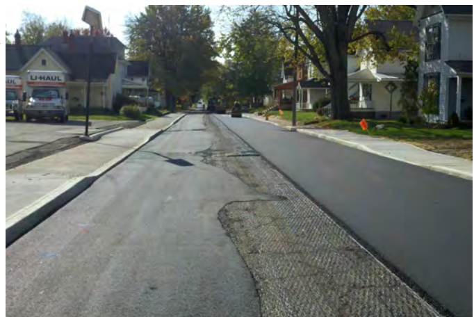
Salamonie Avenue, a Collector Street gets repaved
