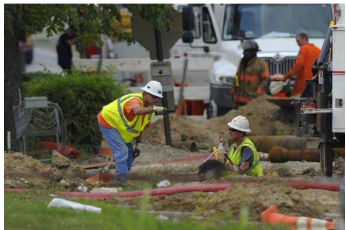
CenterPoint Energy crews upgrade a gas line
