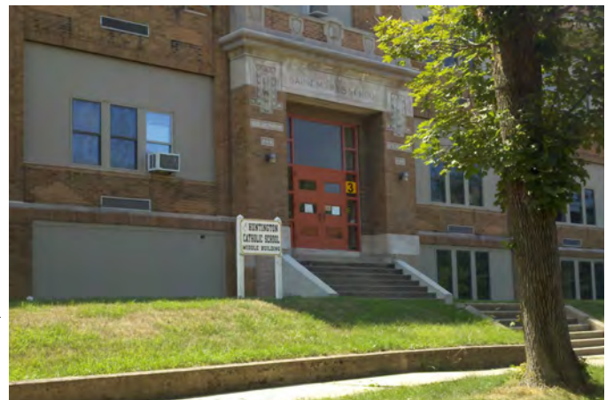
Huntington Catholic School Middle Building
