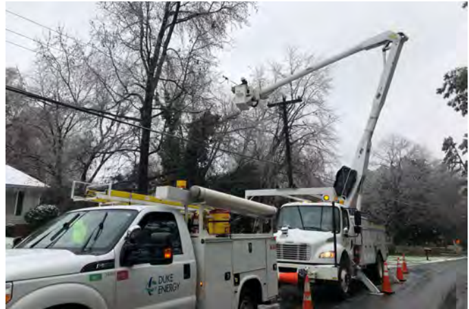
Duke Energy crews repair downed power lines due to ice
