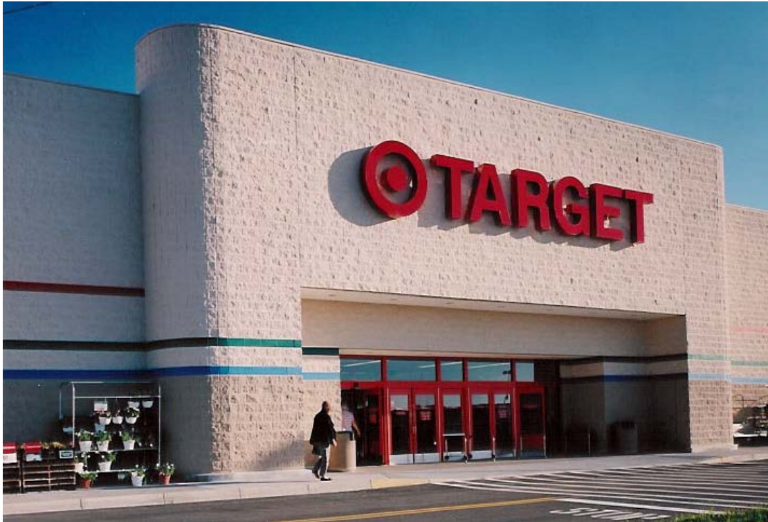
Figure 1: Non-pedestrian scale building
