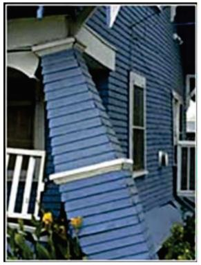
Figure 27 Structural Earthquake Damage
