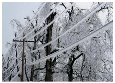
Figure 49 Ice Covered Powerlines
