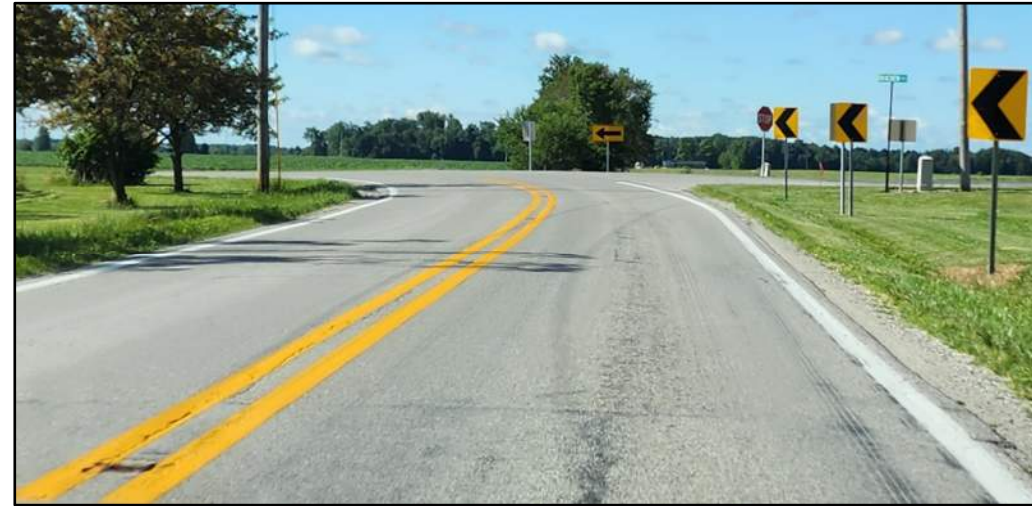
Drivers' view of southbound SR 5 curve at Bracken Rd with 10' travel lanes
