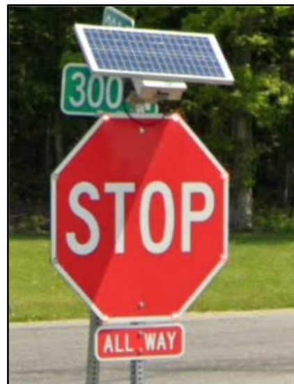
Flashing stop sign at CR 300 E / CR 200 N. The signs were installed after 2 fatal crashes
