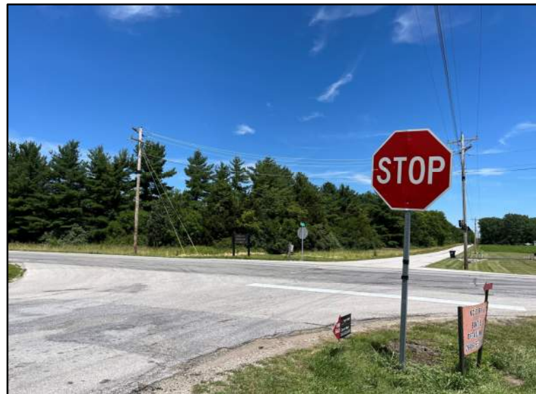
Existing stop sign on eastbound Division Rd at SR 5
