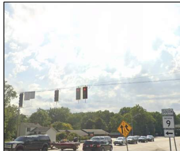
Sunlight glare behind traffic signal for westbound Park Dr
