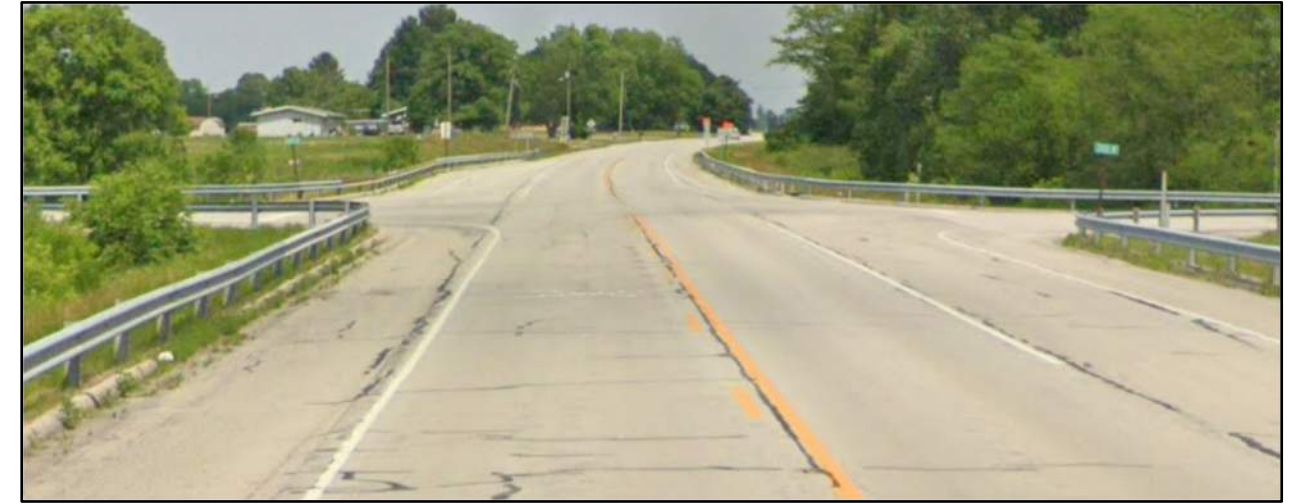
View of CR 300 W intersection from eastbound SR 124
