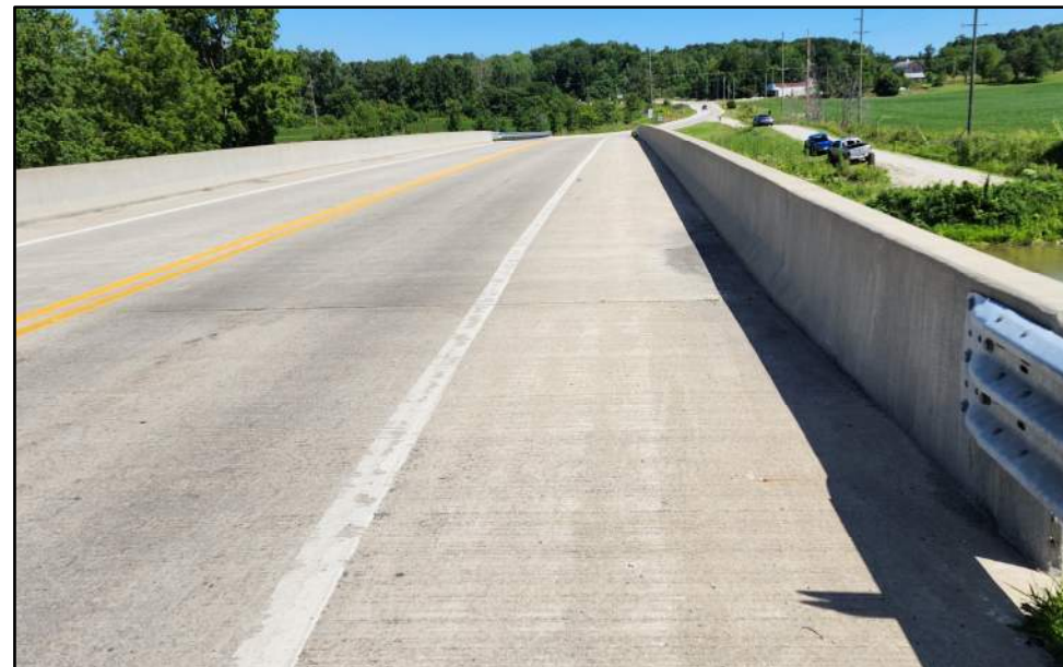
View of northbound shoulder width on SR 105 bridge over Wabash River
