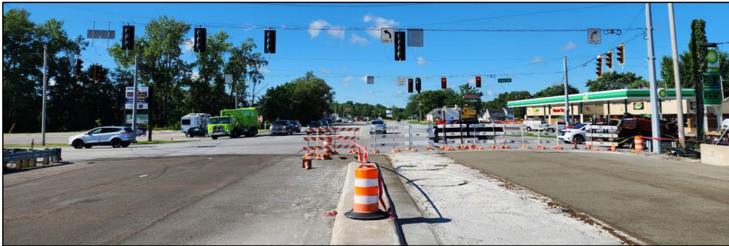
US 24 bridge deck overlay, looking south at CR 900 N intersection
