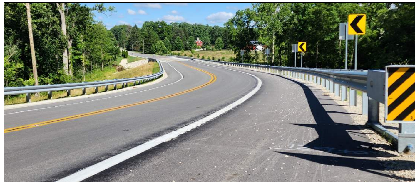
Widened SR 5 bridge and approach over Clear Creek to 12' travel lanes and 5' shoulders, completed in 2023
