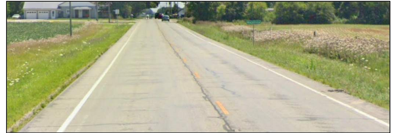
Existing section of SR 5 with 12' travel lanes and 2'-3' shoulders
