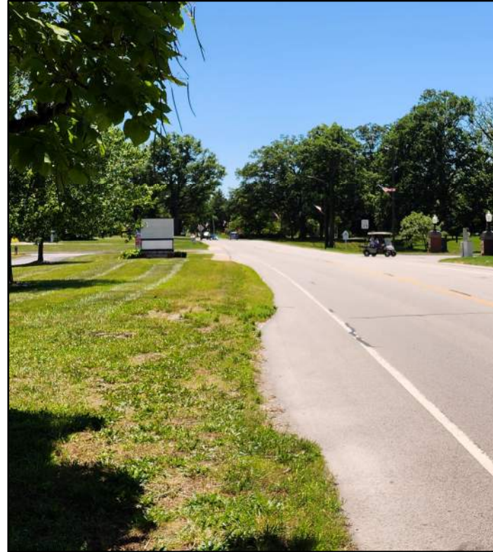
View looking south at end of existing sidewalk
