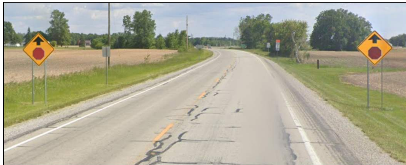
Doubled up stop ahead signs on SR 3 approaching SR 124
