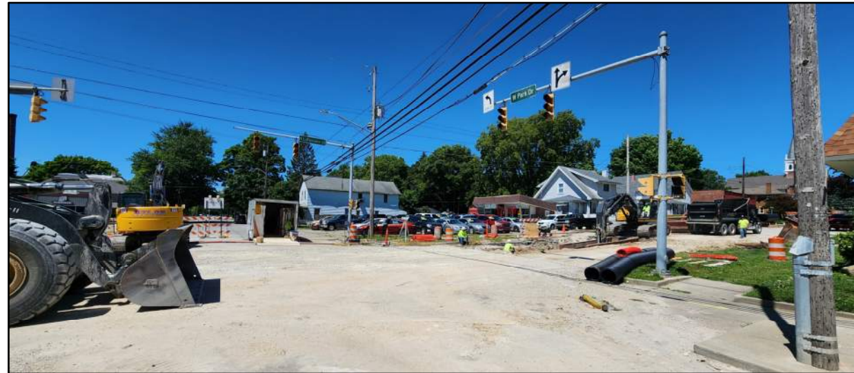
Ongoing reconstruction work at Park Dr / LaFontaine St intersection
