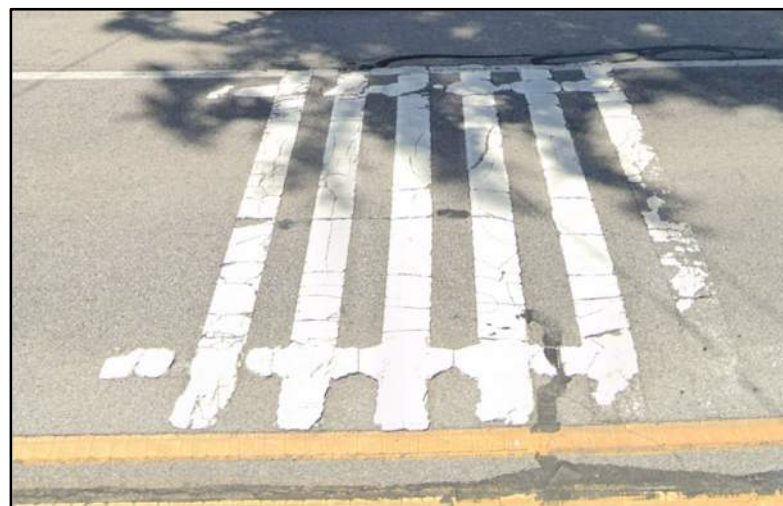
Buzz strips preceding a sharp curve on SR 1 in Leo. There are no known buzz strips in use in Huntington County
