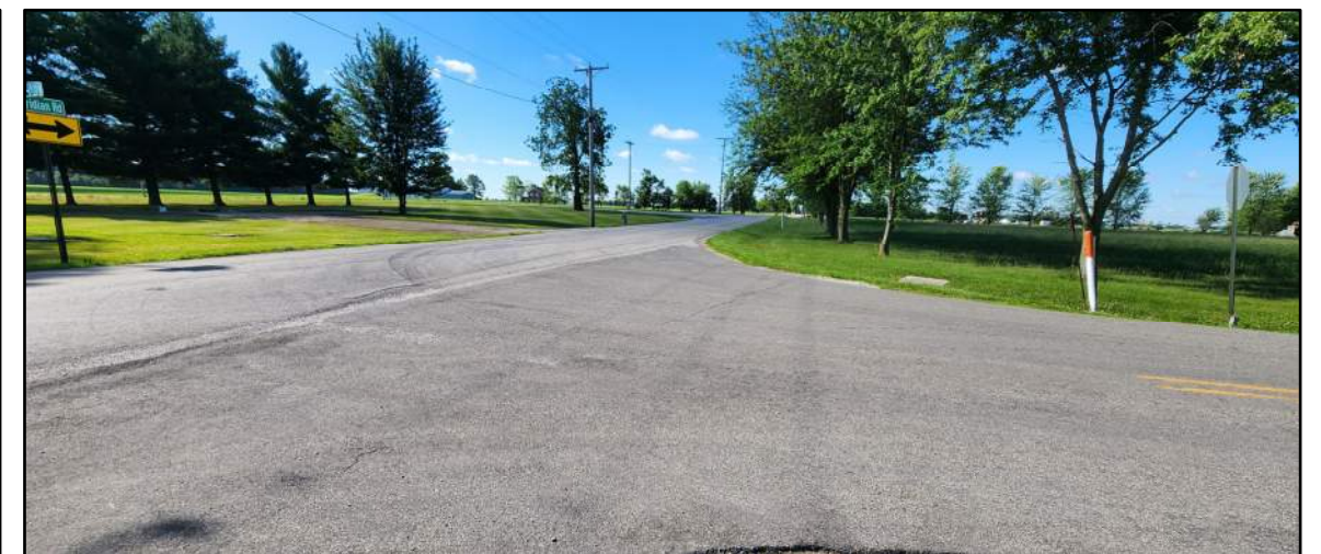
Drivers' view looking south from eastbound CR 900 N at Meridian Rd intersection. Drivers must advance beyond stop sign to gain clear sightlines
