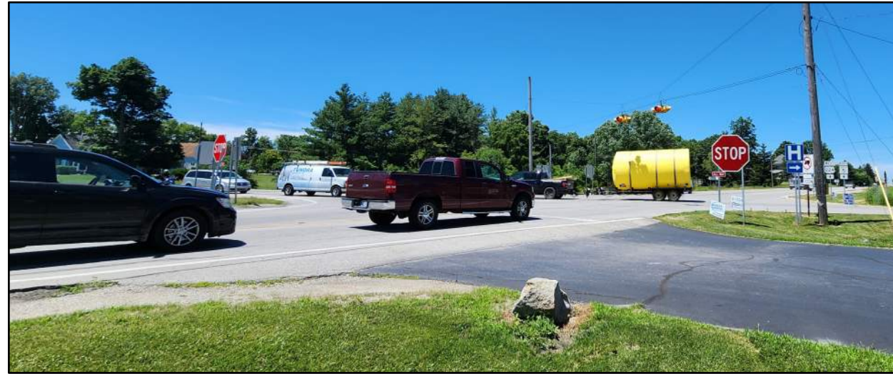
Traffic at US 224 / SR 5 all-way stop-controlled intersection with flashing overhead beacons
