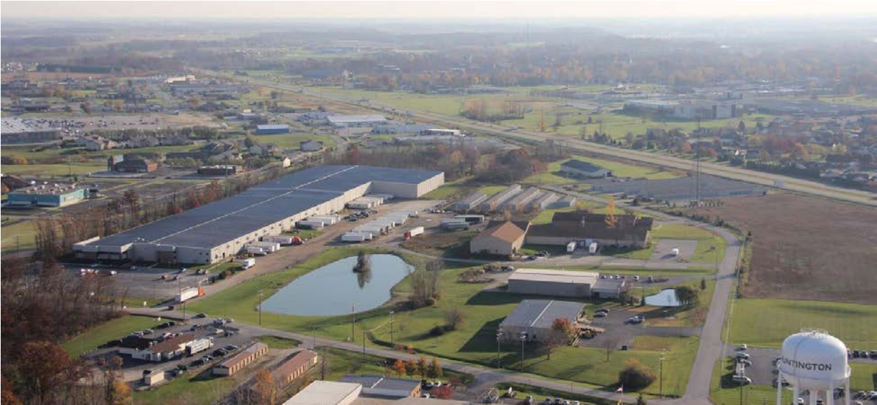
Figure 5-1: Commercial Road Industrial Park has privately-owned acreage available for industrial expansion. Source: HCUED.
