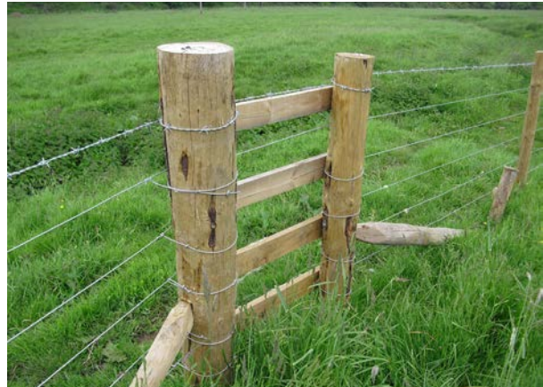
Figure 2-4: An example of fencing suitable for floodplains. Source: www.weadapt.org
